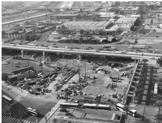
Aerial view of site
