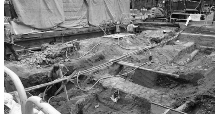
Excavation and utilities support in preparation for deck beam installation
