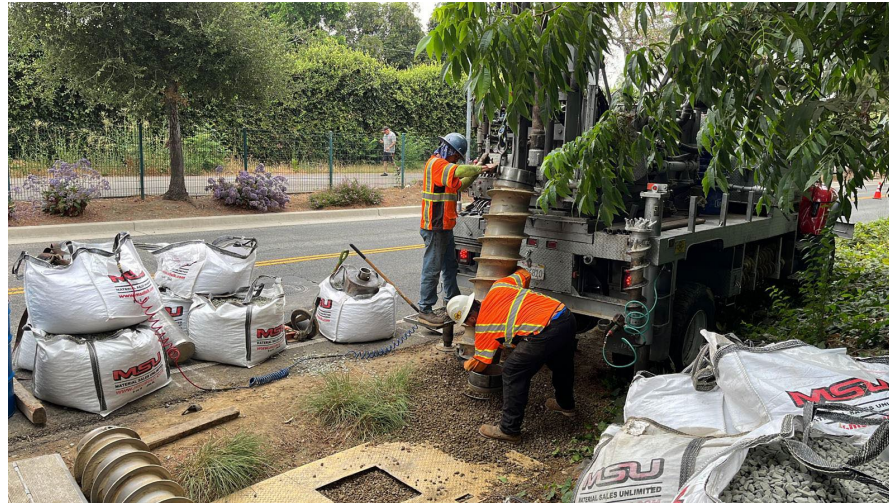
Geotech Infiltration Testing
