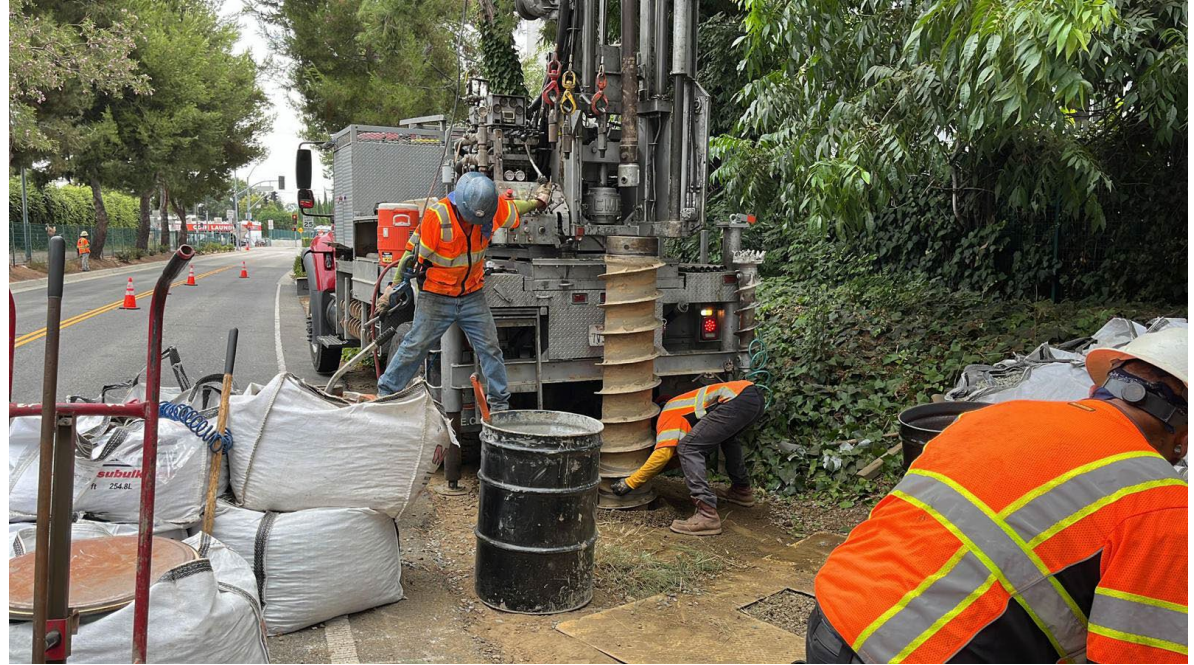
Geotech Deep Infiltration Testing
