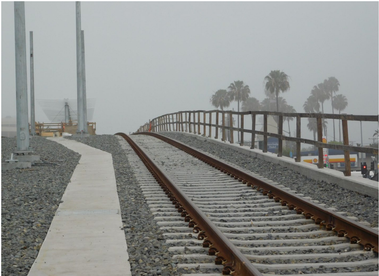
Crenshaw project – K Line - Elevated rail above Aviation Blvd. and W. Century Blvd.
