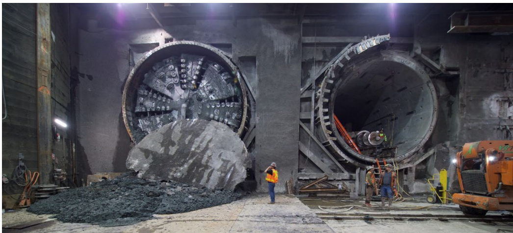
Tunnel Boring Machine break through at Purple Line Extension Section 1
