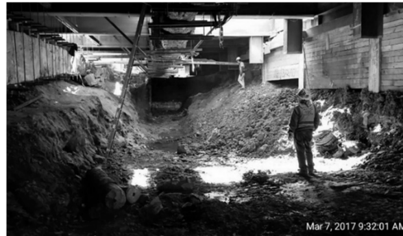
Utility hanging under 2 nd Street decking
