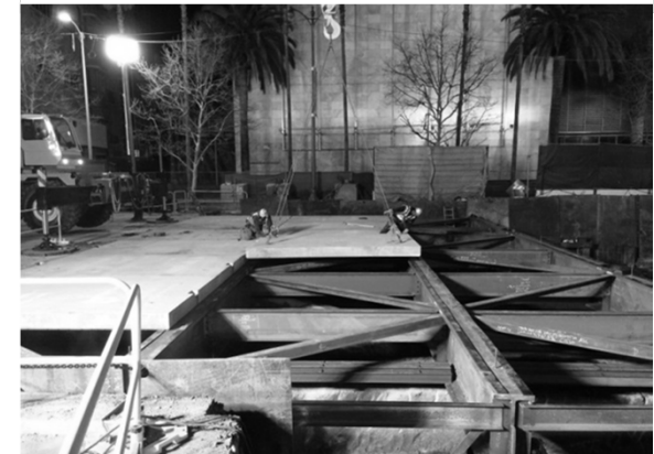
Placement of Deck Panel at Wilshire/Fairfax
