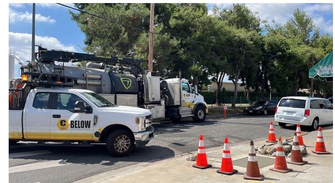
Sidewalk Panel Restoration on Bessemer St
