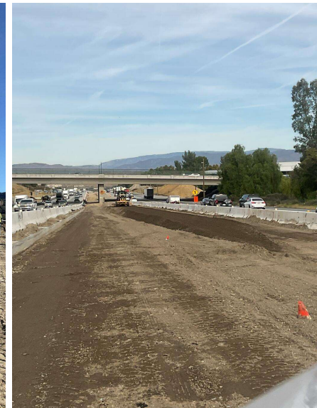
Placement and grading of aggregate base in the median
