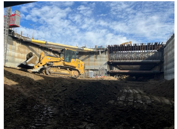
Westwood/VA Hospital Station: Excavation for Level 4 Support
