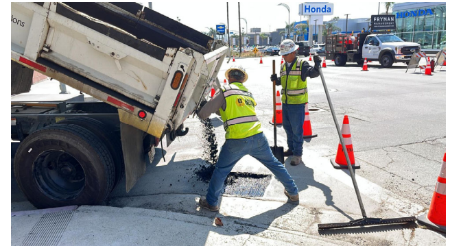
Potholing Restoration on Aetna St
