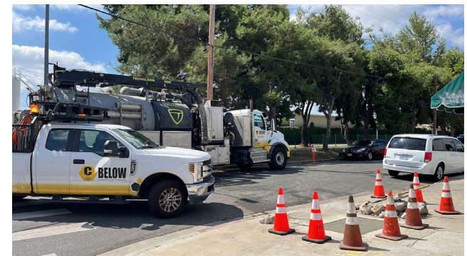
Sidewalk Panel Restoration on Bessemer St
