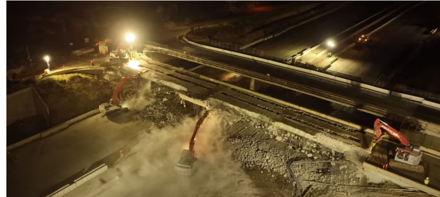
Demolition of old Weldon Canyon Bridge
