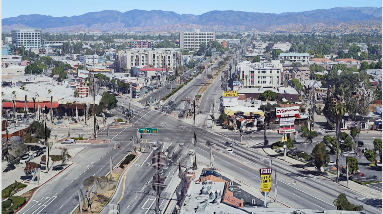
Figure ES-3 – North Hollywood – Vineland Avenue and Lankershim Boulevard Pre-Project
