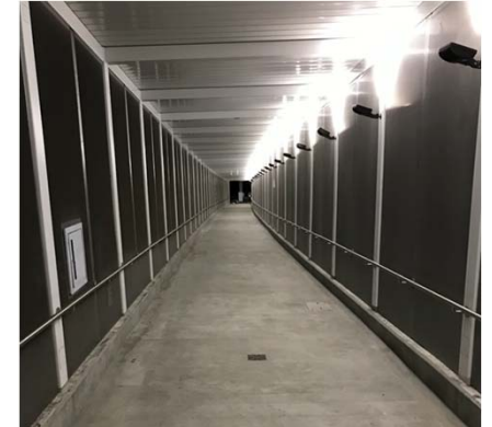
Pedestrian Ramp to Platform
