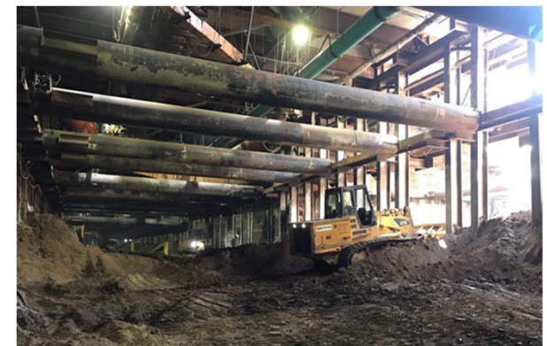
Excavation of the Wilshire/Rodeo Station
