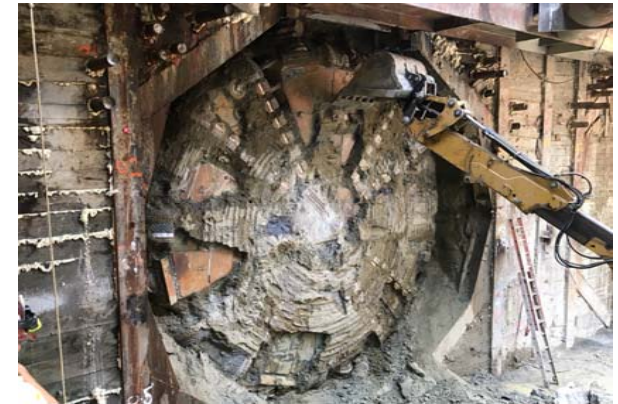
BL TBM "Ruth" at Tunnel Access Shaft
