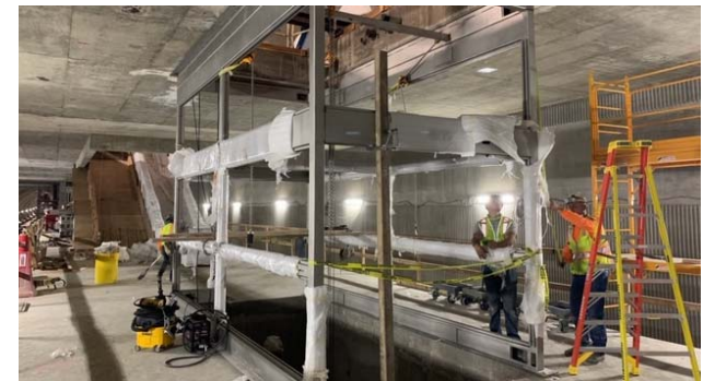
Stainless steel elevator frames at platform level at Historic Broadway Station
