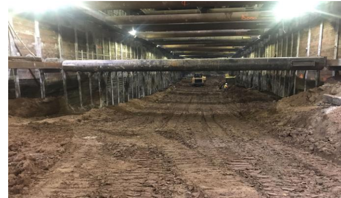
Excavation of the Wilshire/Rodeo Station
