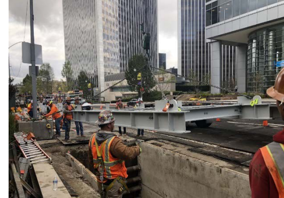
AT&T utility work in Century City
