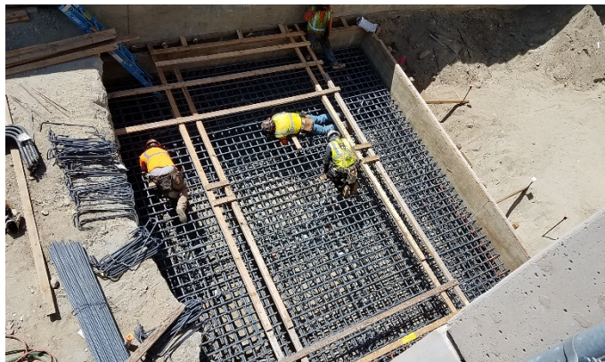
Elevator Footing Forming/Rebar
