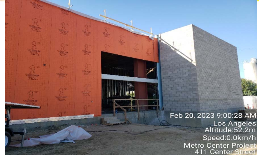
Exterior Finish – Weather Barrier & Sheet Metal
