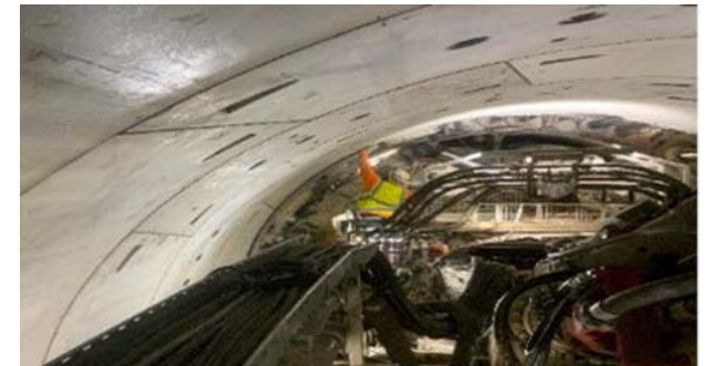
Ring Installation in the BL Tunnel
