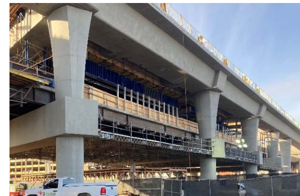
LAWA Station work in progress
