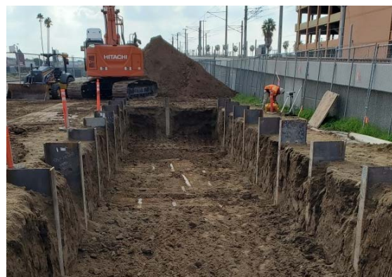
Shoring in progress
