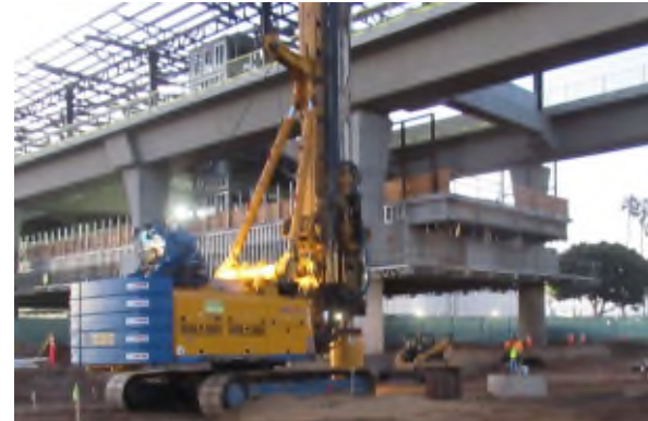
CIDH pile work near APM Station
