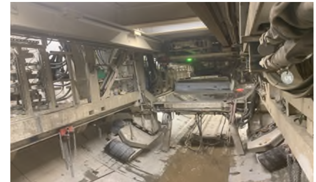
BR TBM Ring Segment Installation
