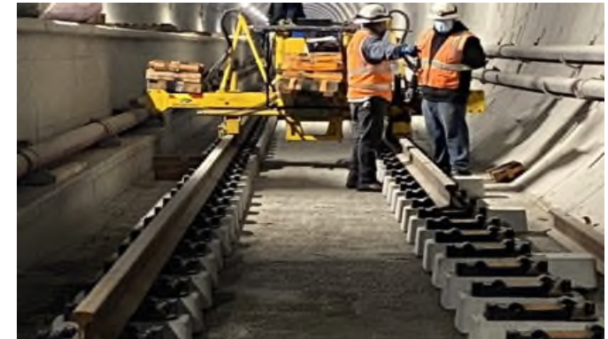
Track Installation in the Reach 1 Tunnel
