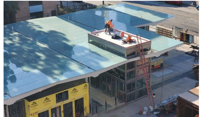
Installation of TPO roofing (Historic Broadway Station)
