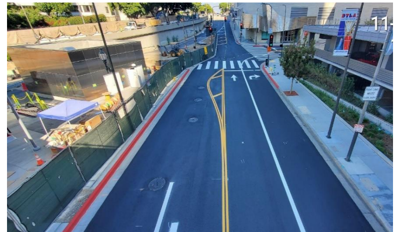
Final asphalt concrete paving along Hope St
