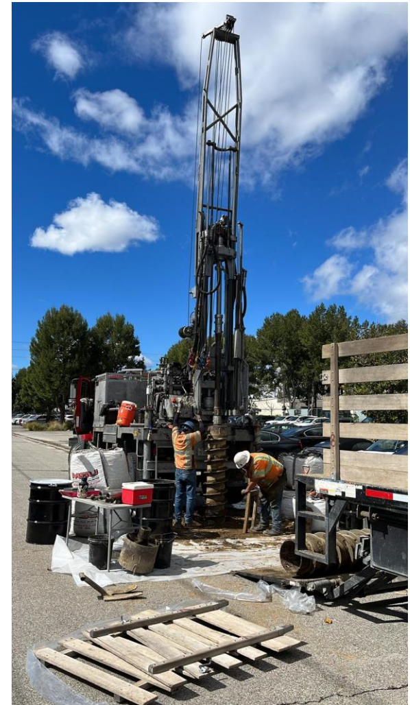
Geotech- percolation testing for stormwater capture scope
