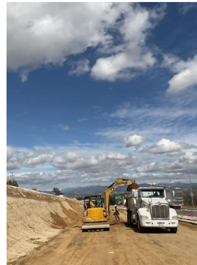
Structural Excavation for RW-2708
