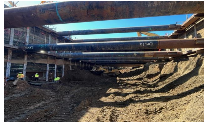
Westwood/VA Station: Excavating station for Level 2 Bracing
