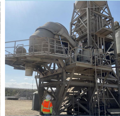
On-site concrete batch plant
