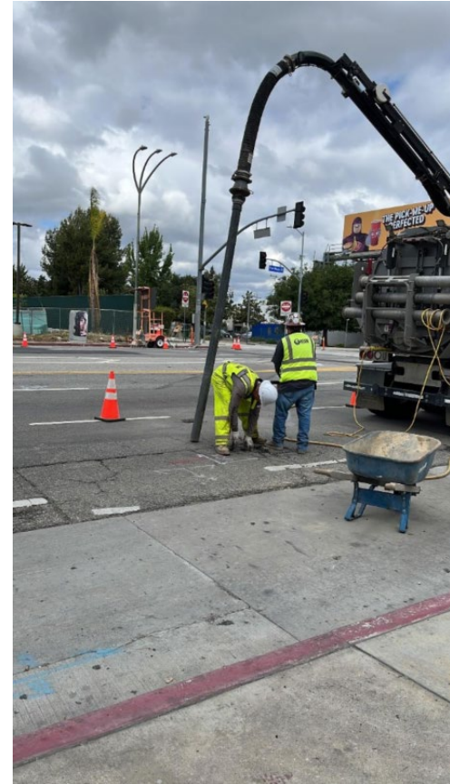
Potholing at Van Nuys Blvd
