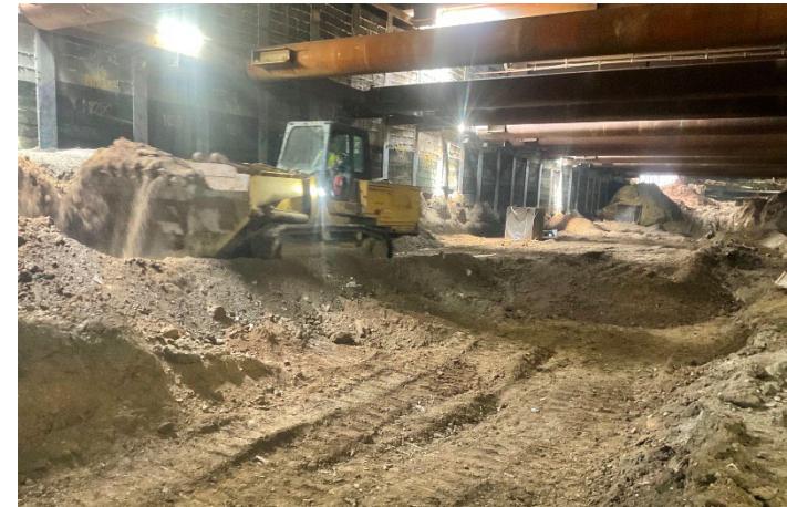
Westwood/UCLA Station: Excavation at Wilshire Blvd
