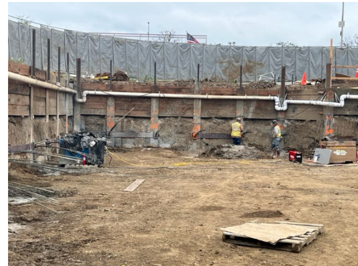
Westwood/VA Station: Tiebacks Installation– North & West Walls
