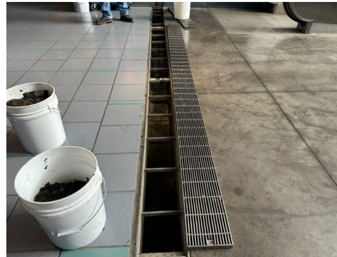
Interior station cleanup to remove debris
