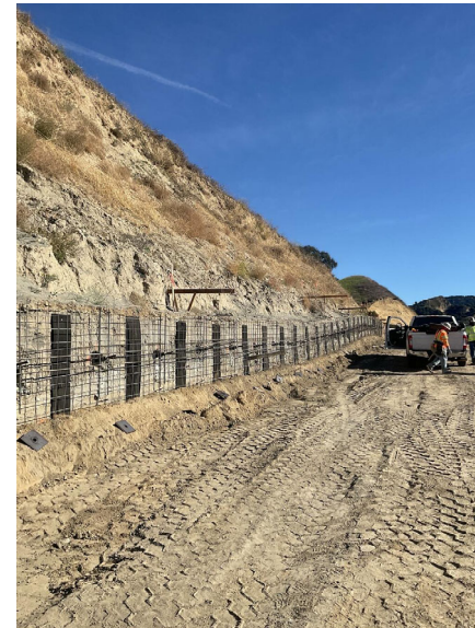
Soil nail installation at Retaining Wall 2524
