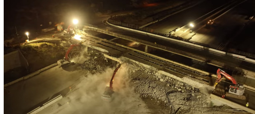
Demolition of old Weldon Canyon Bridge
