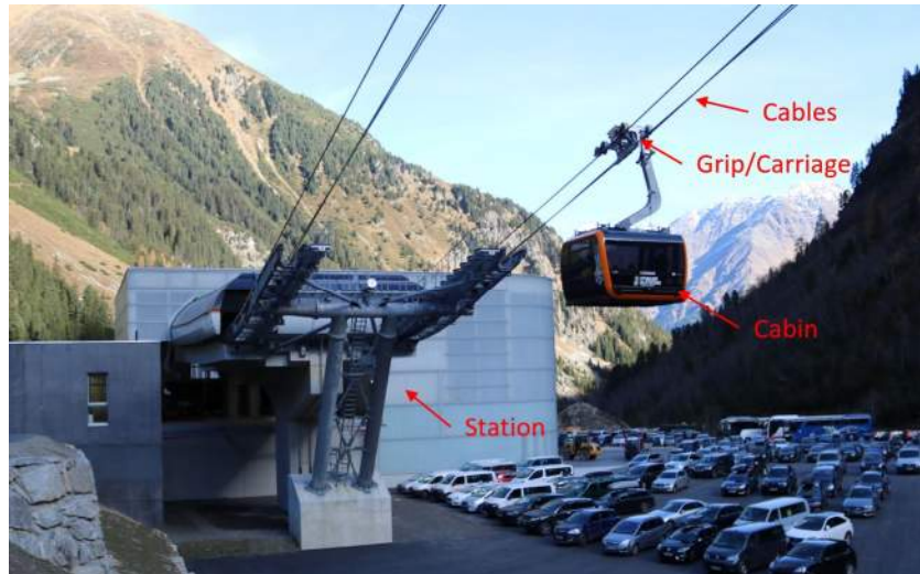
Image 2 – Components of a 3S Gondola System
