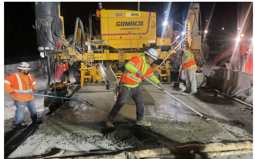
Jointed Plain Concrete Paving in Median
