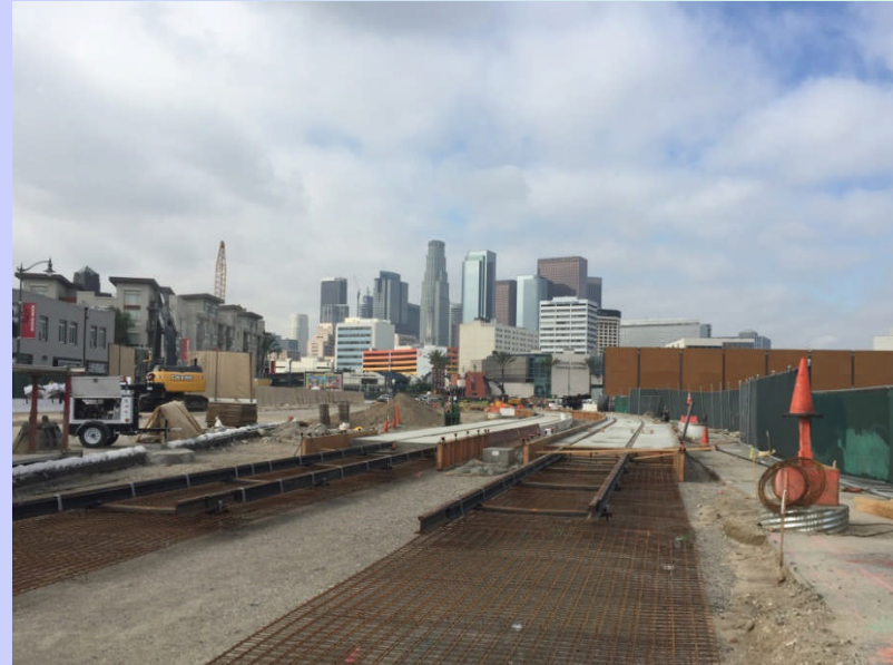
Shoofly installation at Mangrove Yard
