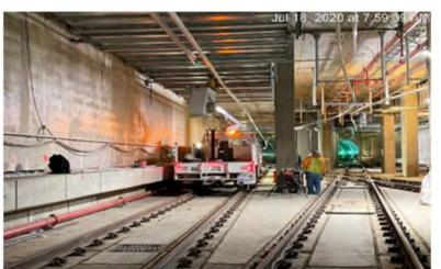
Continue installing supports and fixtures for the crossover lighting at the invert level of Expo/Crenshaw
