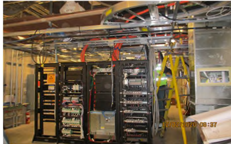
Leimert Park Station – contractor working on communication rack in train control and communication room.
