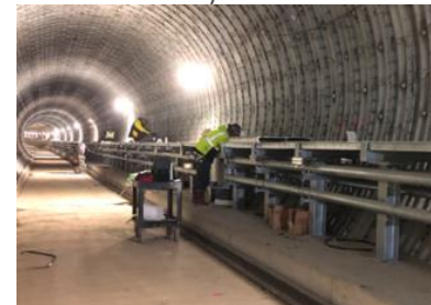
Tunnels: Steel Walkway Construction BL Tunnel
