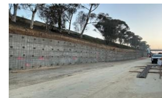
105WB RW 270 Soil Nail Wall Exterior
