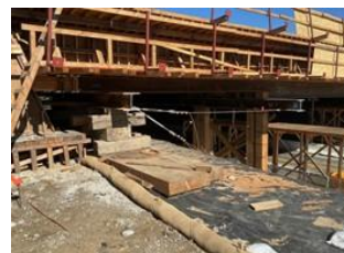
105EB Stanford bridge falsework
