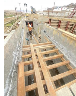
Drain System 406 Formwork Install
