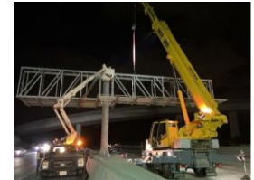
Sign Structure Truss Installation
